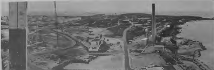
AT LEFT is part of eastern tankfarm area with NFAR unit. At right is Seron Colorado residential area with Powerhouse No. 2 in foreground.
